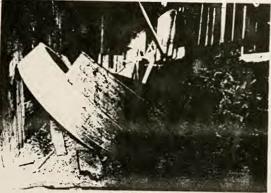
Figure 96. Revenue Mill (structure #34) interior of upper level showing wooden fly wheels that drove stamps.
